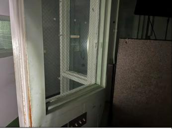
Photo 12 – Test 36, greater than 1 mg/cm<sup>2</sup> lead containing light green paint on metal window frames in 111 bldg.
