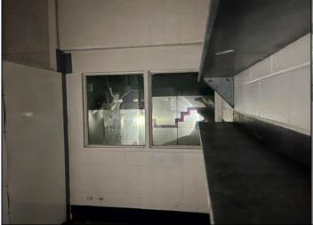
Photo 11 – Test 35, greater than 1 mg/cm² lead containing white paint on metal window frames in 111 bldg.
