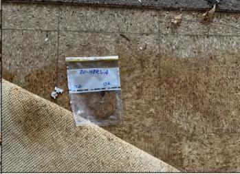
Photo 4 – Sample 311-HBRS-A, 3% asbestos containing black mastic on 9" brown floor tile in the 109 building. Only the mastic contains.
