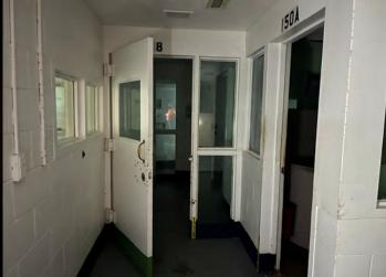
Photo 10 - Tests 15, 23, 25, 26, and 33, greater than  $1 \text{ mg/cm}^2$  lead containing white paint on metal doors and door frames in 111 bldg.
