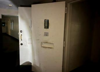
Photo 9 – Tests 15, 23, 25, 26, and 33, greater than 1 mg/cm<sup>2</sup> lead containing white paint on metal doors and door frames in 111 bldg.
